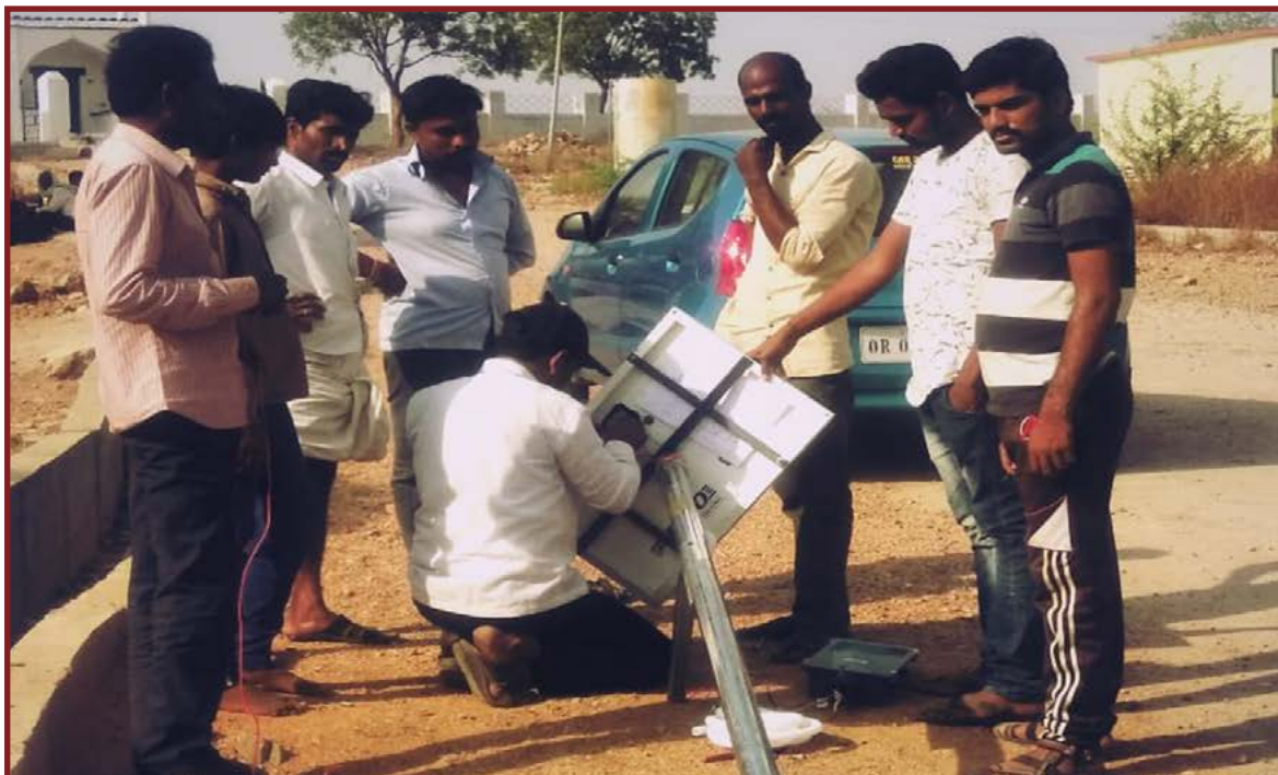
Installation of solar street lights at village
